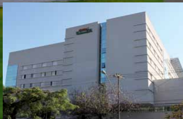
Hospital Unimed Belo Horizonte, Brasil
