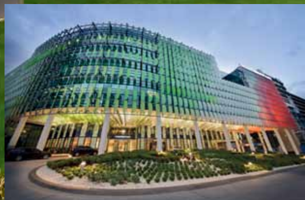
The Royal Children's Hospital, Melbourne, Australia
